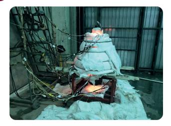
The objective of the solution annealing in the field is to promote the dissolution of precipitated carbides at high temperature followed by rapid cooling, so that these elements remain in solid solution.
